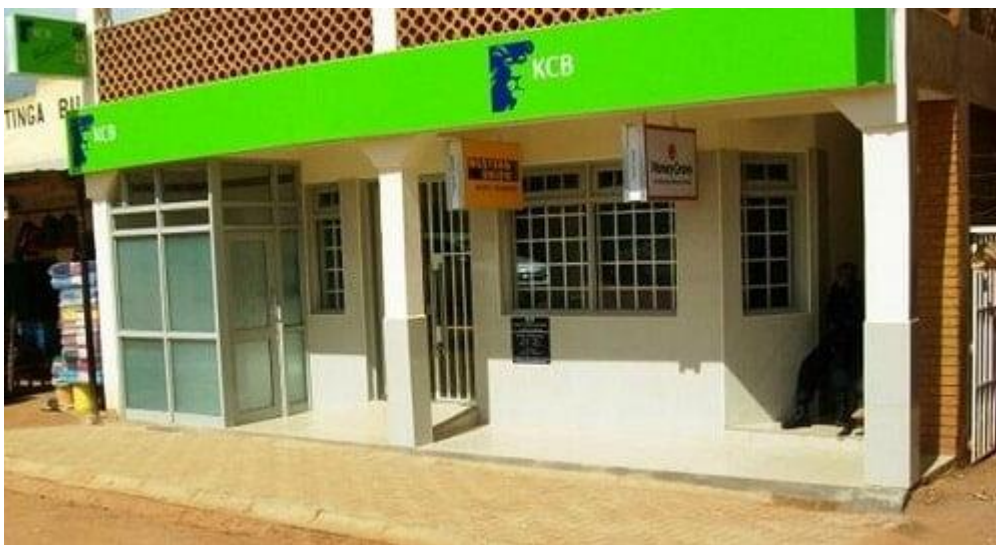
Figure 6 Kenya Commercial Bank -Ugunja Branch
