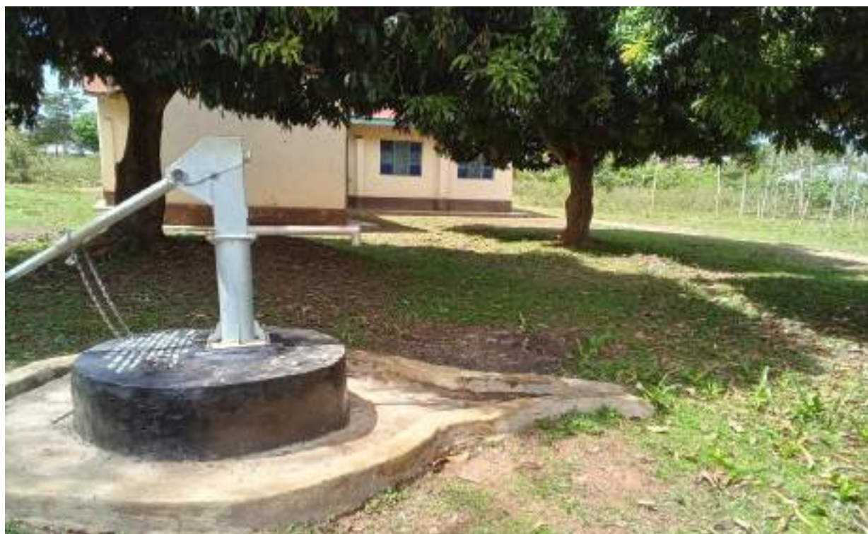
Plate 3-15: A borehole in Komolo area within Siaya Municipality
