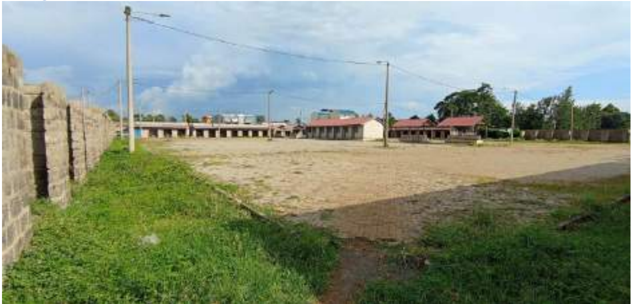
Plate 3-41: Bus Terminus under Construction
