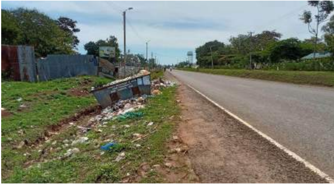
Plate 3-19: Poor solid waste management along a section of Luanda- Siaya Road
