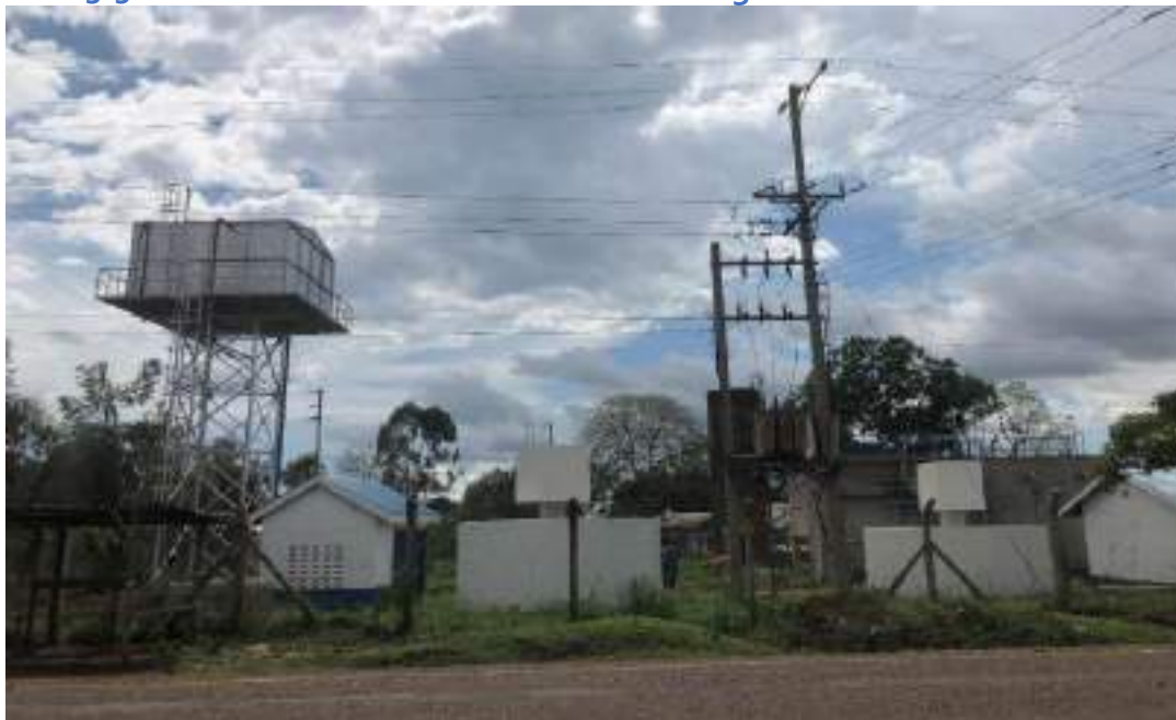
Plate 3-52: SIBOWASCO Treatment Plant in Mbaga Area
